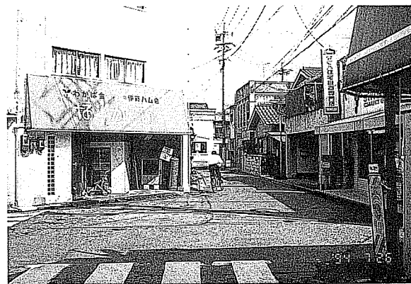
写真 24 神辺宿川北の遠見遮断部分 (1994.7.26) The Crossroad to Obstruct the View from a distance at Kawakita in Kannabe
